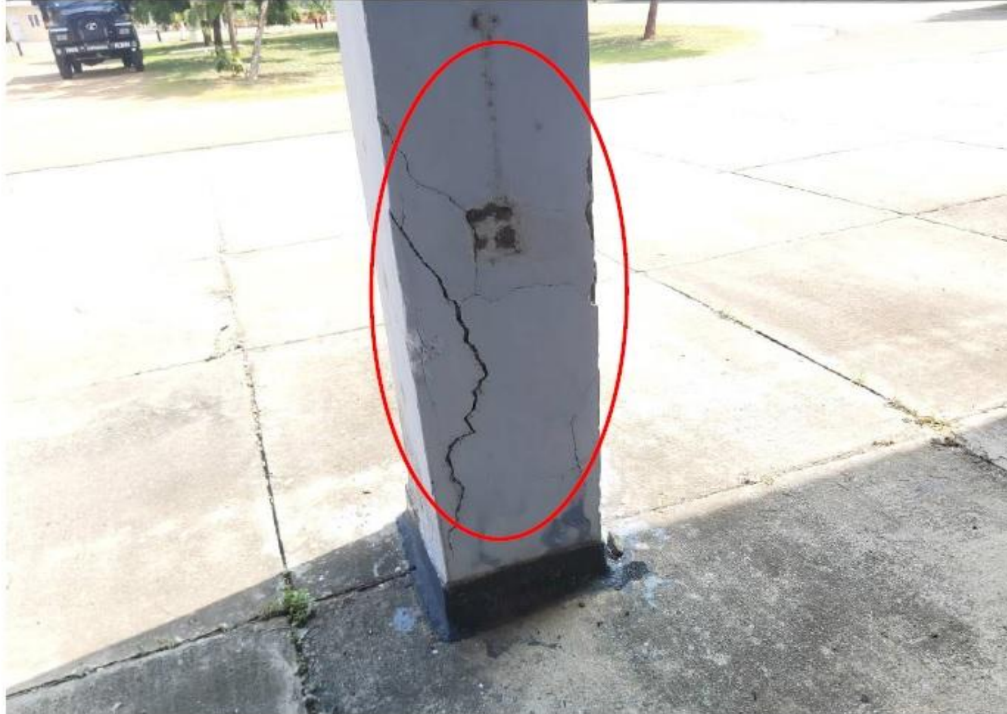
Photo 2 A view of the cracking in a RC column A3 at the front side of the garage
