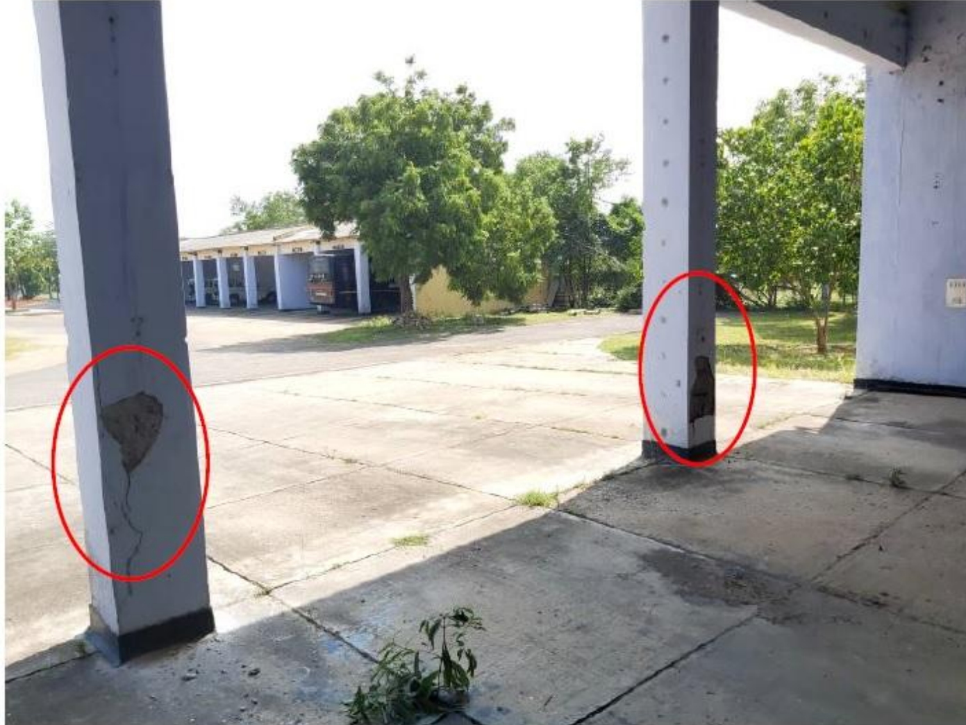
Photo 4 A view of the spalling of concrete and exposure of rebars in the RC columns A6 & A7 at the front side of the garage
