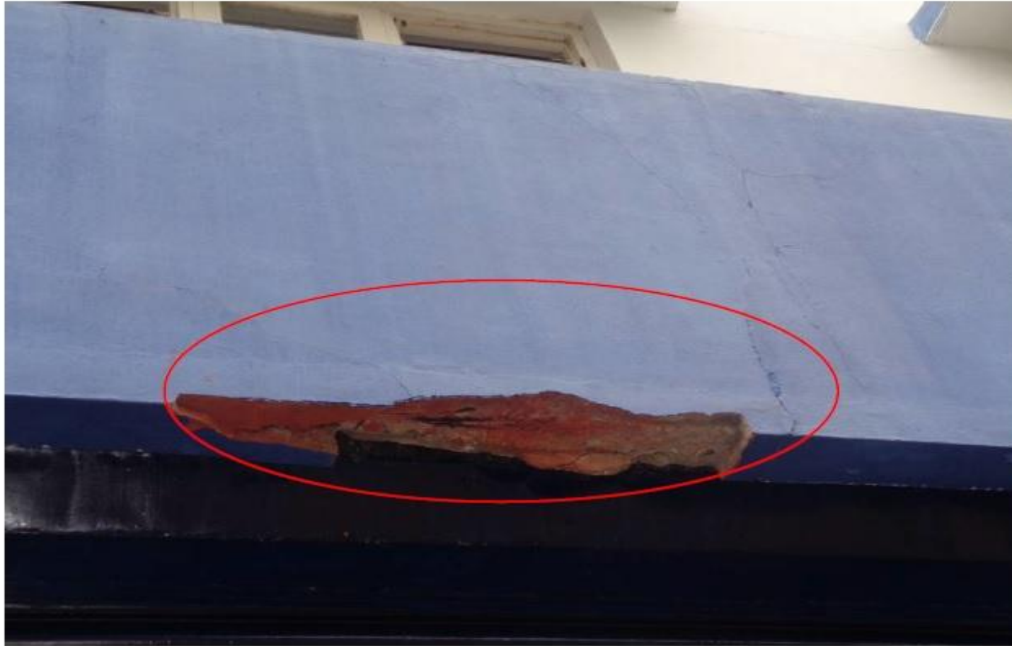
Photo 2 A view of the cracking and spalling of concrete in the RC drop panel at the front side of the building
