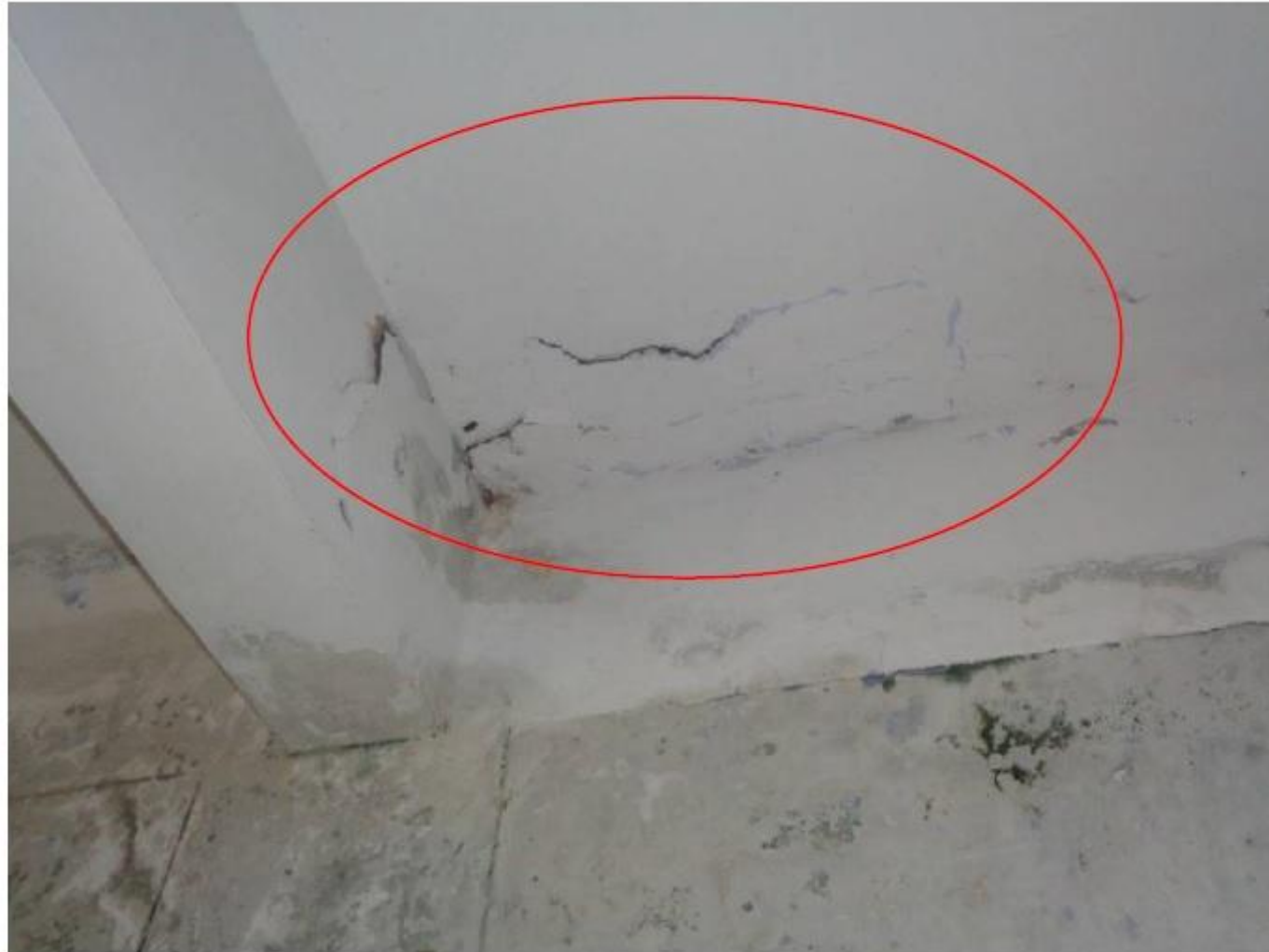
Photo 10 A view of the cracking in the RC slab of the passage area in the first floor
