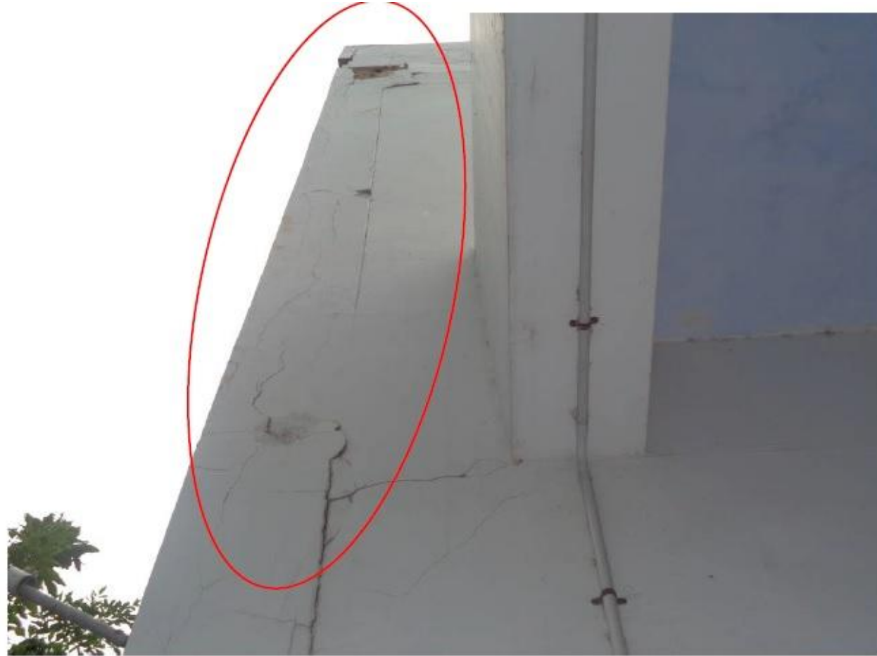
Photo 3 A view of the cracking and spalling of concrete in the RC column D7 at the exterior face of the building
