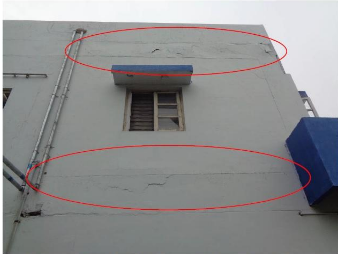
Photo 4 A view of the cracking in the RC beams at the exterior face on the North-west side of the building
