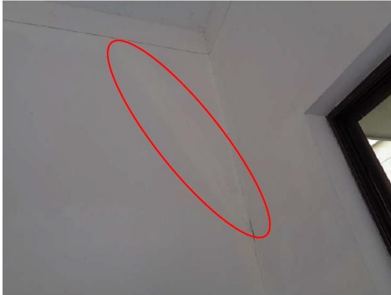
Photo 5 A view of the cracking in the masonry wall at the reception area at the interior of the building
